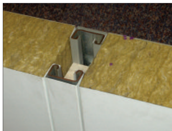
Figure 17: Insulated core panels – internal
